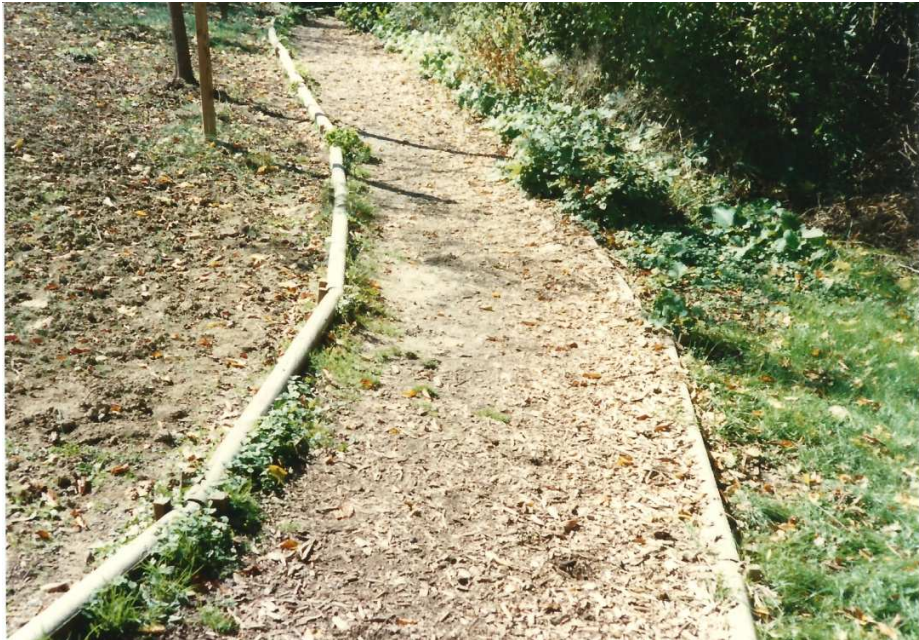
A wood chip trail surface, Brooks Nature Center, Olgebay Institute, Wheeling, W.VA.
