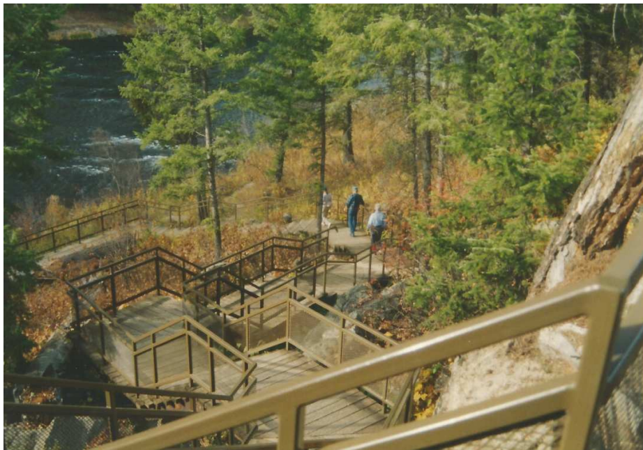
Stairway connecting the upper and lower loops of the Mesa Falls Trail, Targhee National Forest. Note the absence of railing once the boardwalk is on the ground (by the visitors in the Photo) Photo courtesy of the Targhee National Forest, Ashton, Idaho.
