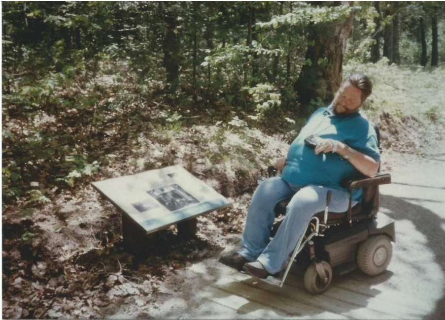
Trail user Scott McDonald on the Maywood History Trail, Little Bay de Noc Recreation Area, Manistique Ranger District, Michigan. The trail is 4 feet wide with a maximum slope of 5%. It uses a lay and limestone mixture for the trail tread and has rest benches spaced every 2-- feet. The wooden slats are located by interpretive stops. (Photo courtesy of Manistique Ranger District).
