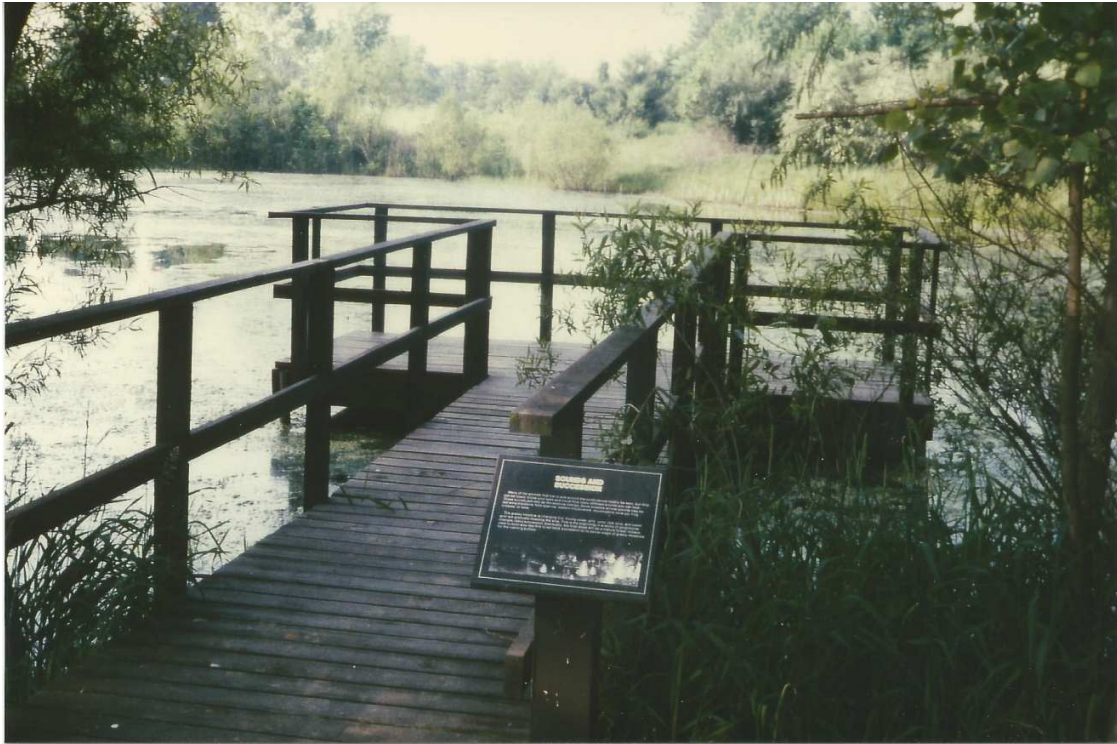
Viewing deck with interpretation, Carlisle Lake (a Corps of Engineers park), Illinois.
