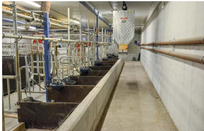
The feeding table for the tie stalls allows individual feeding of roughage. Concentrates are given in separate mangers.
