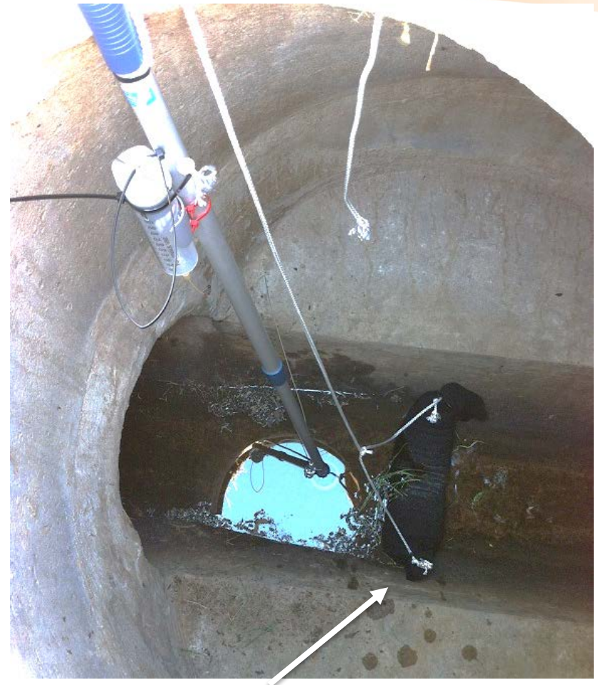
Dam to increase water height (Jeans leg with sand)
