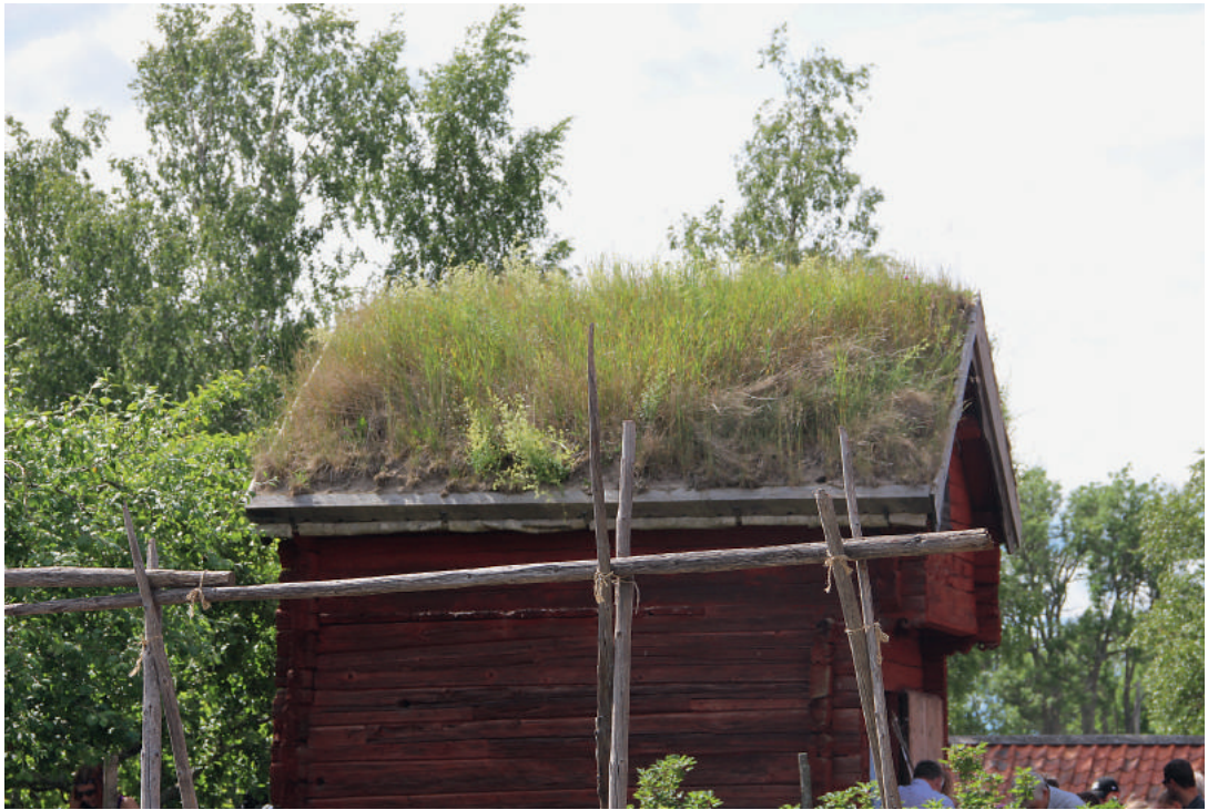
FIGURE 4. Reconstructed green roof on one of the wooden buildings in the Disagården open-air museum in Uppsala. PHOTO: Maria Ignatieva, 2015.
