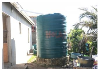
Photo 1. Rainwater tank attached to downpipe from the tin roof in Manteku. Purchases of rainwater tanks have increased with the access to cash transfers and local savings groups in these villages
