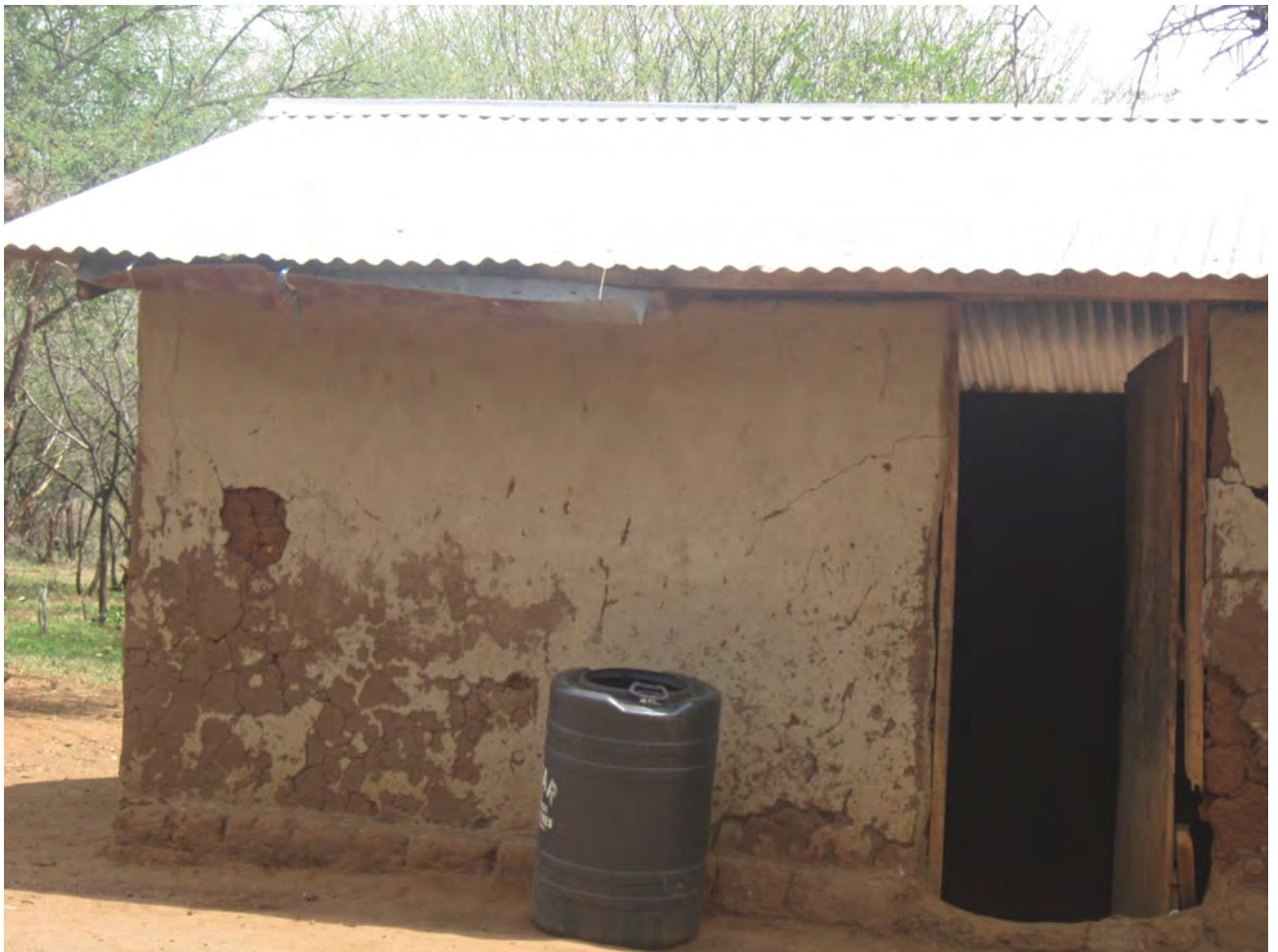
Fig. 54: Example of roof-top water harvesting where the pipe under the roof collects water and drives it into a container (M. Virginia Bile, June 2023).
