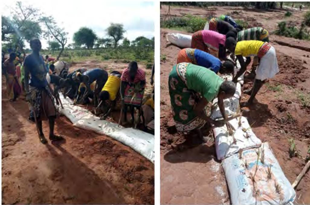
Fig. 7: Women planting vetiver grass on the sacks laid along a contour line in June 2022 at the LC (Nyaga M.N., 2022b).
