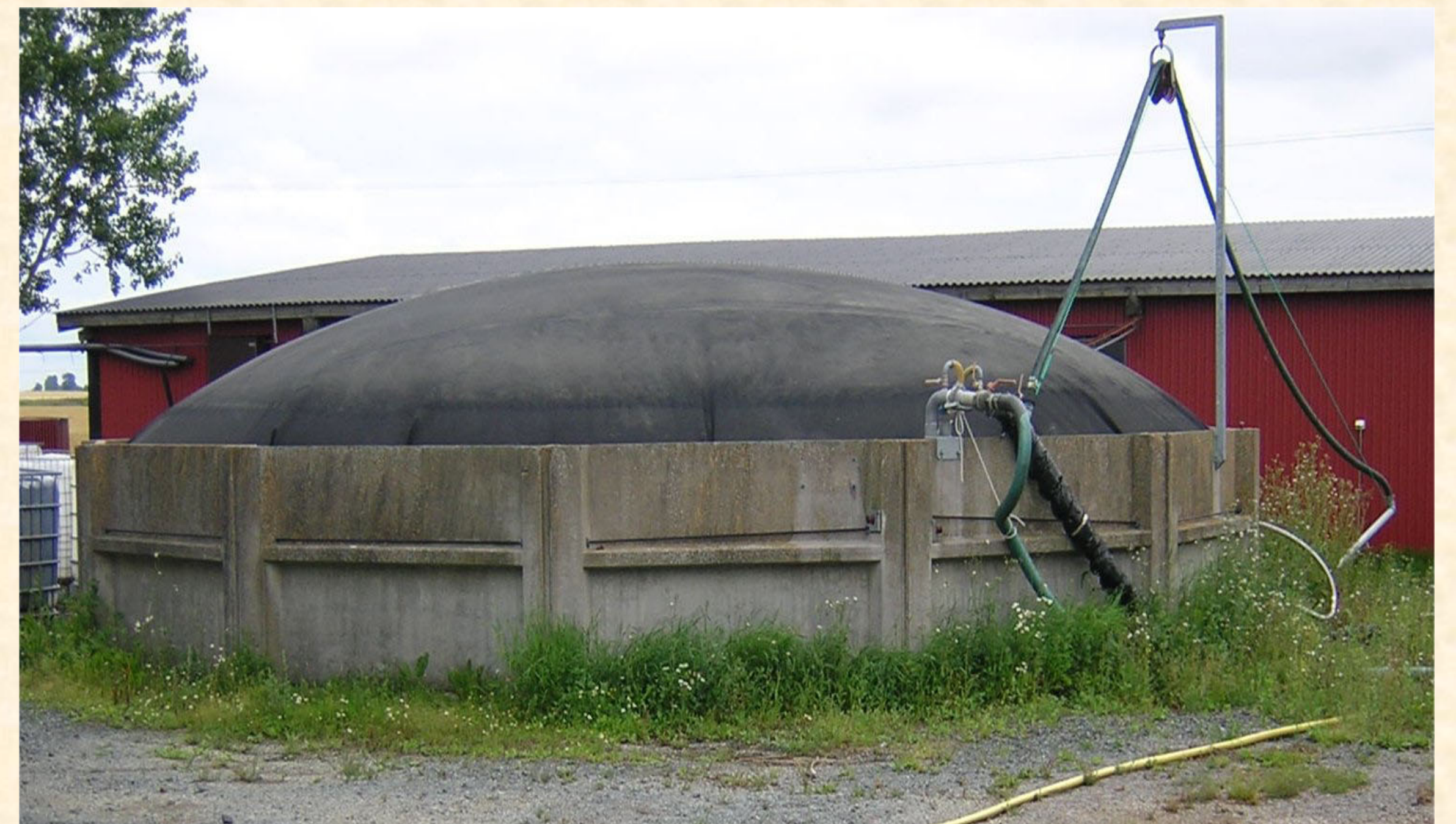
Experimental stirred reactor tank for one-step biogasification. Estimated methane yield was 0.21 \text{ m}^3 \text{ kg VS}^{-1} .
