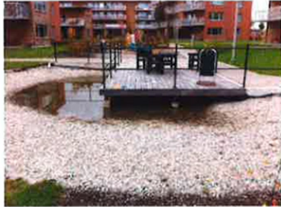
Area 2 uses visible solutions with canals and ponds (similar to those in Augustenborg) to manage rainwater. The pictures show examples of how this system can look.
