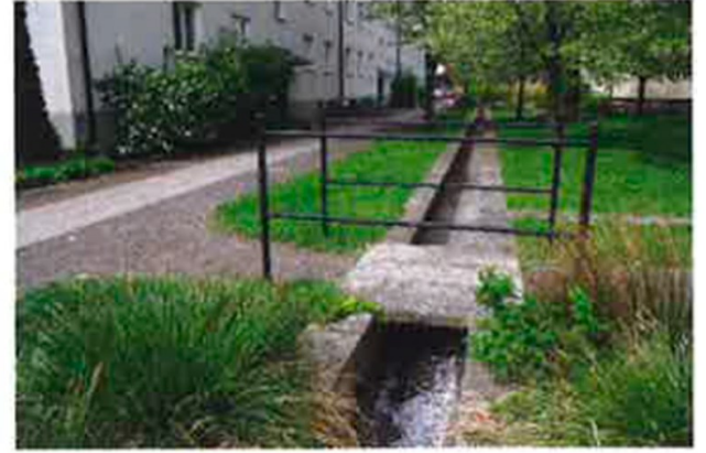
Area 2 uses visible solutions with canals and ponds (similar to those in Augustenborg) to manage rainwater. The pictures show examples of how this system can look.
