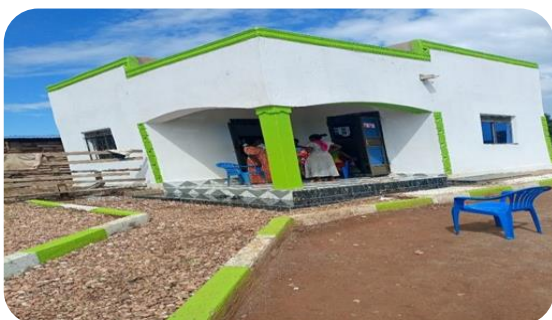
Kinoni Milk processing facility
