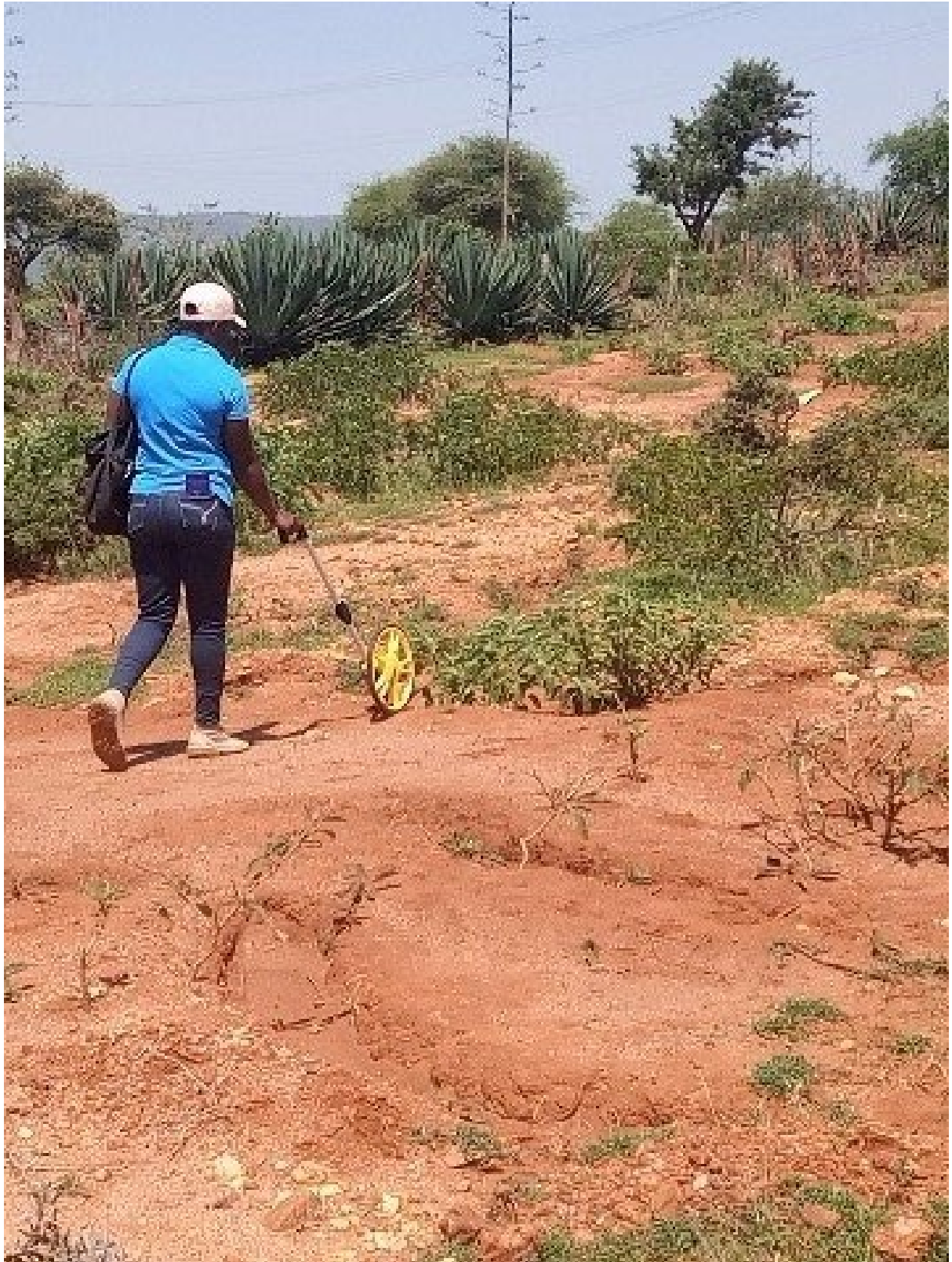
Margeret Nyaga is measuring the gully to be rehabilitated. Photo: Stephen Mureithi
